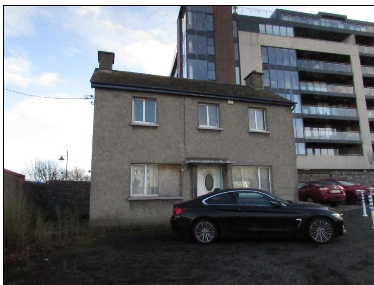
Figure 4. Photograph of the 2-storey building at the site. Image taken 02/12/2020.
